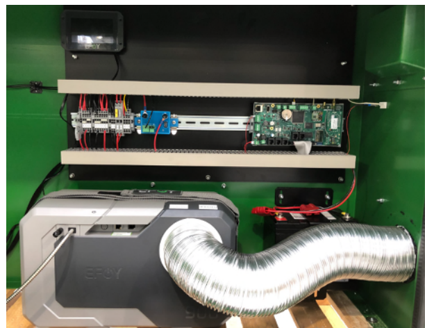
Inside a flood detection cabinet
