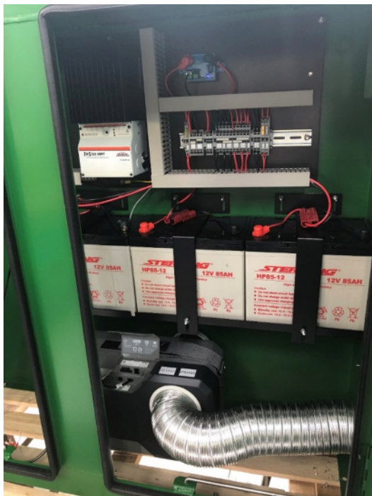
Inside a control cabinet
